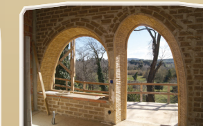
Earth bricks and clay plaster support and improve breathing
