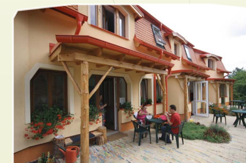
The finished house, the place for the spirit of the Self of man...
